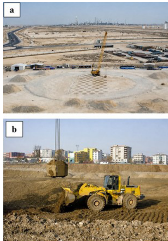
Figure 6. Ground improvement procedure using dynamic replacement in soils: (a) Site with Dr columns; (b) Crawler bulldozer filling the columns. Zetas (2015).
