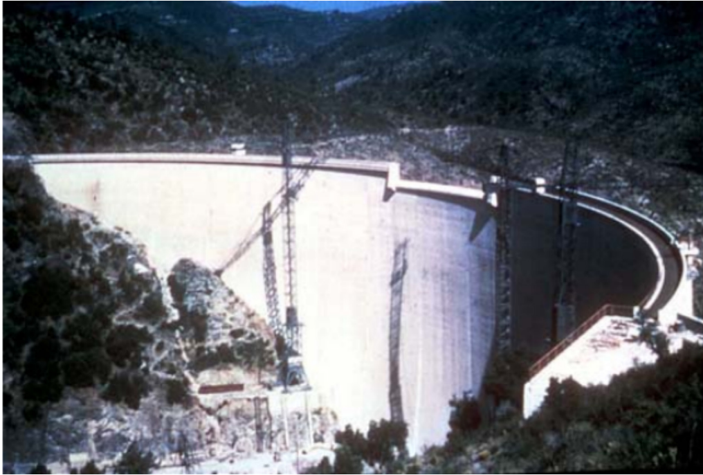
Figure 4. Photo of Malpasset dam at the end of the construction (photo from Coyne and Bellier, in Duffaut, 2011). The construction started in April 1952 and was completed two years later, in October 1954, say 5 years before the accident.
