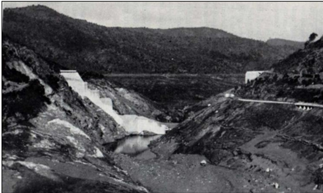
Figure 11. Photo of the dam after the accident on 2nd December, 1959 (Mary, 1968 in Duffaut, 2013a).
