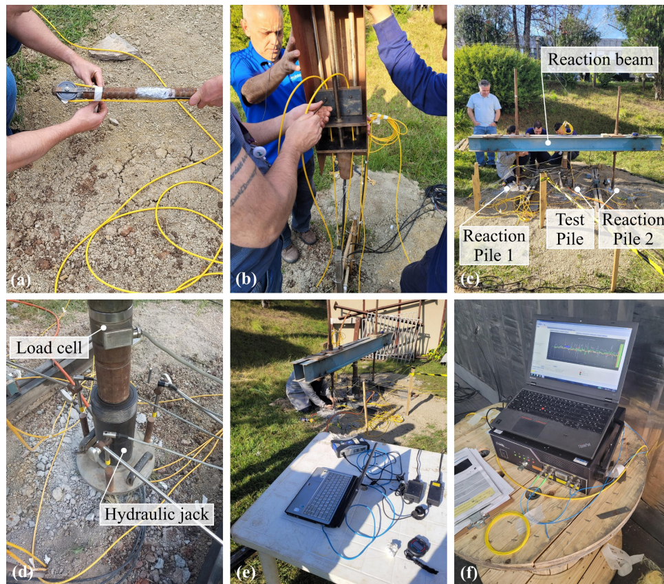
Figure 2. Experimental setup of the fiber optic instrumentation and static load test: (a) pulley at the pile tip, (b) system for fiber pre-tensioning, (c) general assembly of the static load test, (d) detail of the test pile head – load cell and hydraulic jack, (e) data acquisition system, and (f) DSTS OzOptics interrogator.
