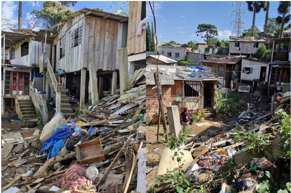
Figure 2. Built Structures in the “Portelinha” Community, Curitiba, Brazil.
