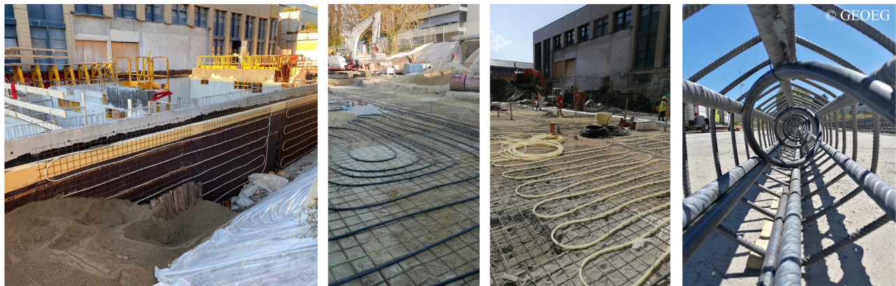
Figure 1. Installation of heat exchanger tubes on reinforcement cages of foundation structures before pouring concrete or integrated into drainage paths (image source: GEOEG, 2025).
