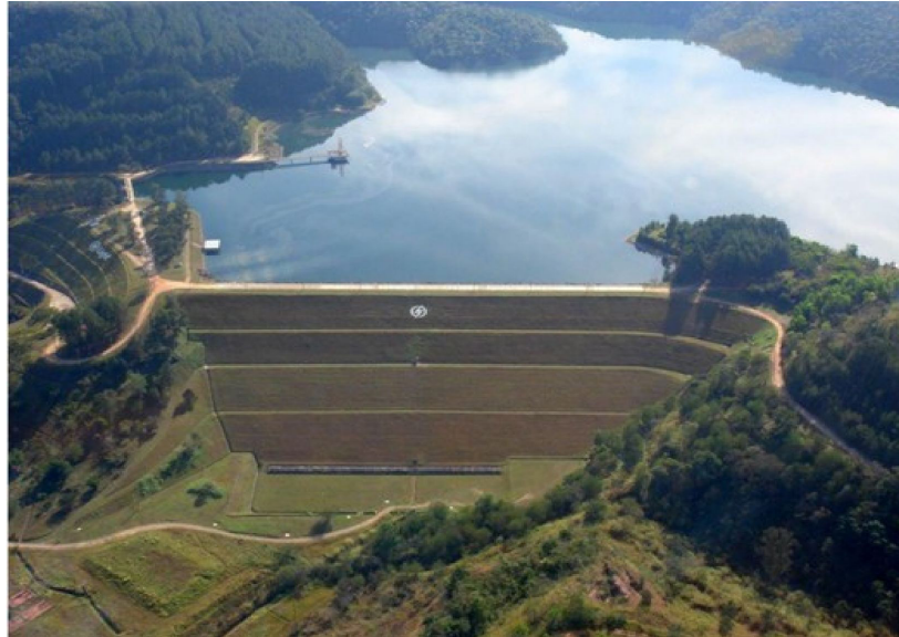
Figure 6. Santa Branca Dam. Aerial view of the downstream slope in mid-2017 (Araújo & Sayão, 2018).
