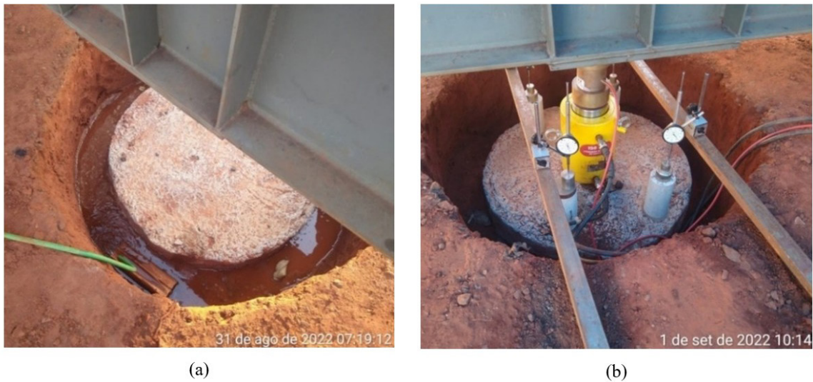
Figure 3. Load test on isolated footing with soil in flooded state: (a) Pre-flooding of soil; (b) Water flow ceased and test started.
