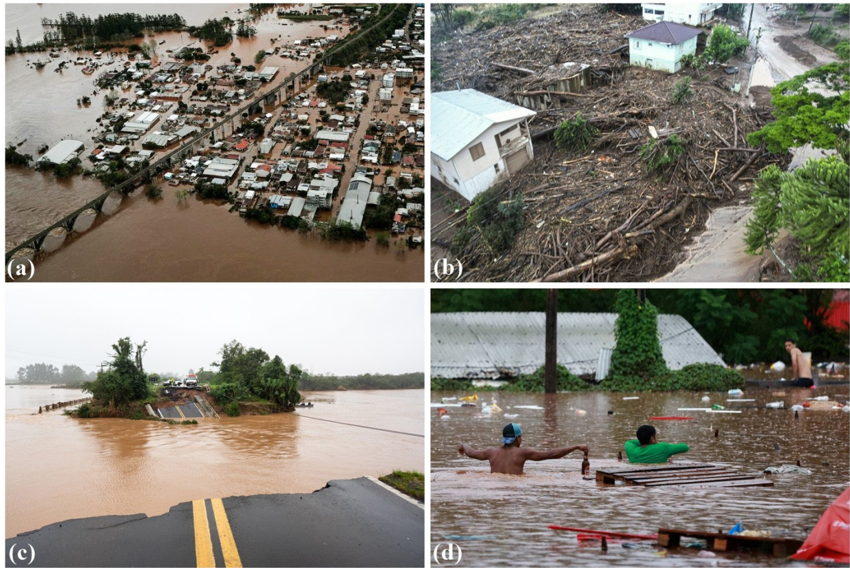
Figure 1. Documented geotechnical impacts from 2024 Rio Grande do Sul floods: (a) urban flooding (2.8 m depth, Porto Alegre) (Gonzatto, 2024); (b) landslide (12,000 m 3 displacement, Serra Gaúcha) (Estadão Conteúdo, 2024); (c) bridge collapse (4.2 m scour depth, Eldorado do Sul) (Pinheiro, 2024), and (d) residential inundation (18-23 days) (Fuhrmann, 2024).
