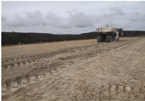
Figure 17. Example of cement mixing of a pulverised chalk.
