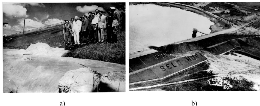
Figure 2. High-risk inspection conducted at the Pampulha Dam, Belo Horizonte (CMBH, 1954): (a) expert group; (b) rupture of the dam.
