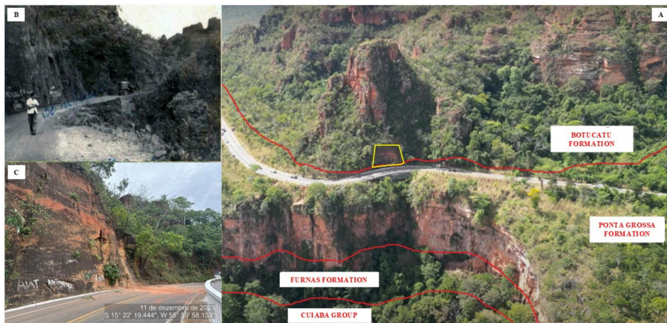
Figure 3. Gravitational mass movement of the rockfall type on highway MT 251 in the Chapada dos Guimarães region, in the State of Mato Grosso, Brazil. (a) Photo of the site before the construction of the viaduct in 1959; (b) Detail of the rock mass in 2023; (c) General view of the Portão do Inferno area in 2023.
