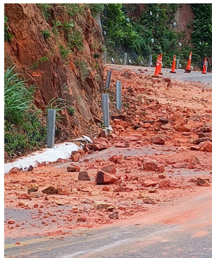
Figure 8. Rock blocks fallen over the highway as a validation of the mapping work (Conciani, 2024).
