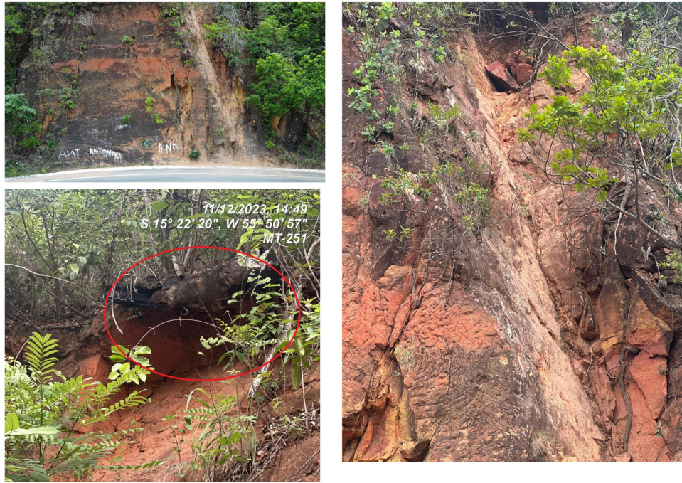
Figure 4. Examples of unsupported blocks in a wedge rupture scar following a fall related to the lower layer of the sedimentary rock (Conciani, 2024).
