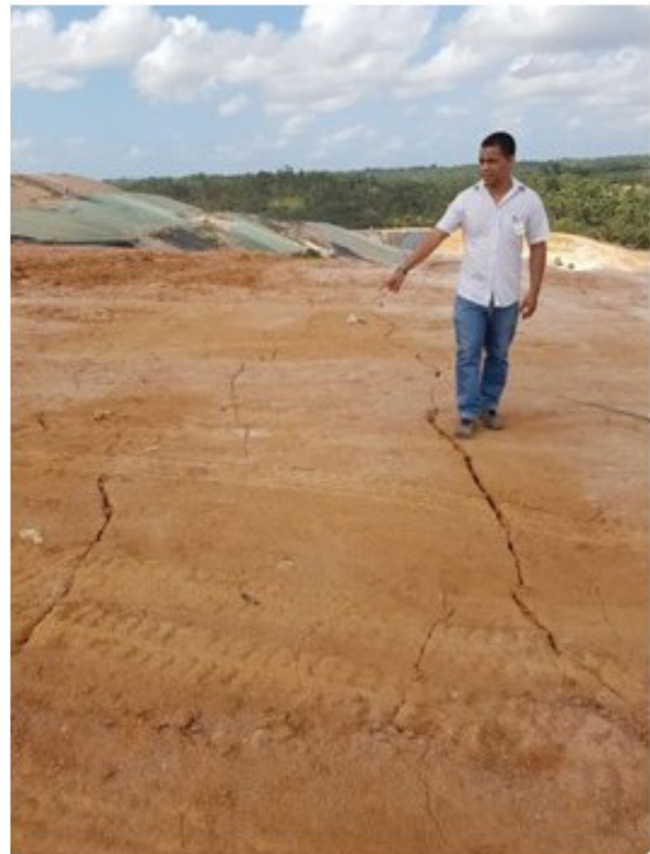
Figure 2. Cracks development in the contact between two waste uplifting with different ages.
