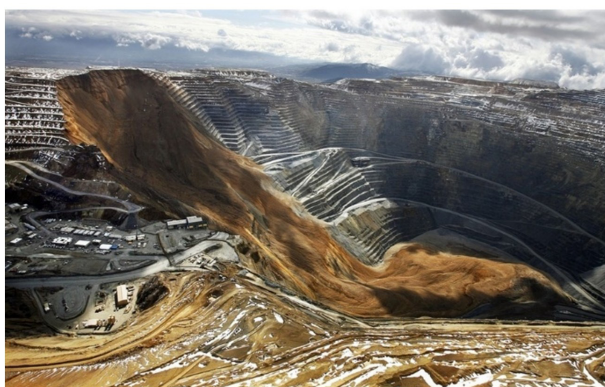
Figure 8. Landslide at the 1.2 km deep Kennecott Copper Bingham Canyon open pit mine (Geoengineer, 2013).
