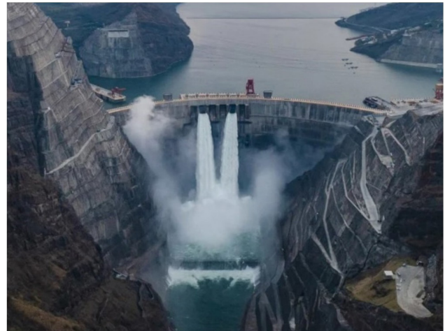
Figure 4. Baihetan mega-dam with two open spillways (Chik, 2023).
