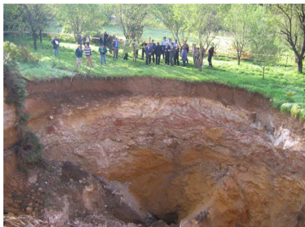
Figure 9. Chimney break in a closed gypsum mine (Didier et al., 2008).
