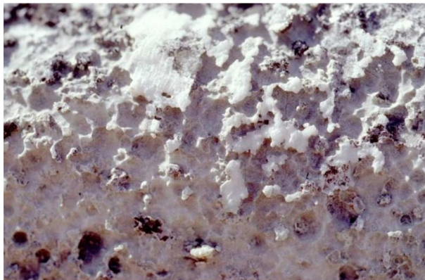
Figure 12. Biocolonisation on limestone of the Jerónimos Monastery in Lisbon (Delgado Rodrigues, 2007).
