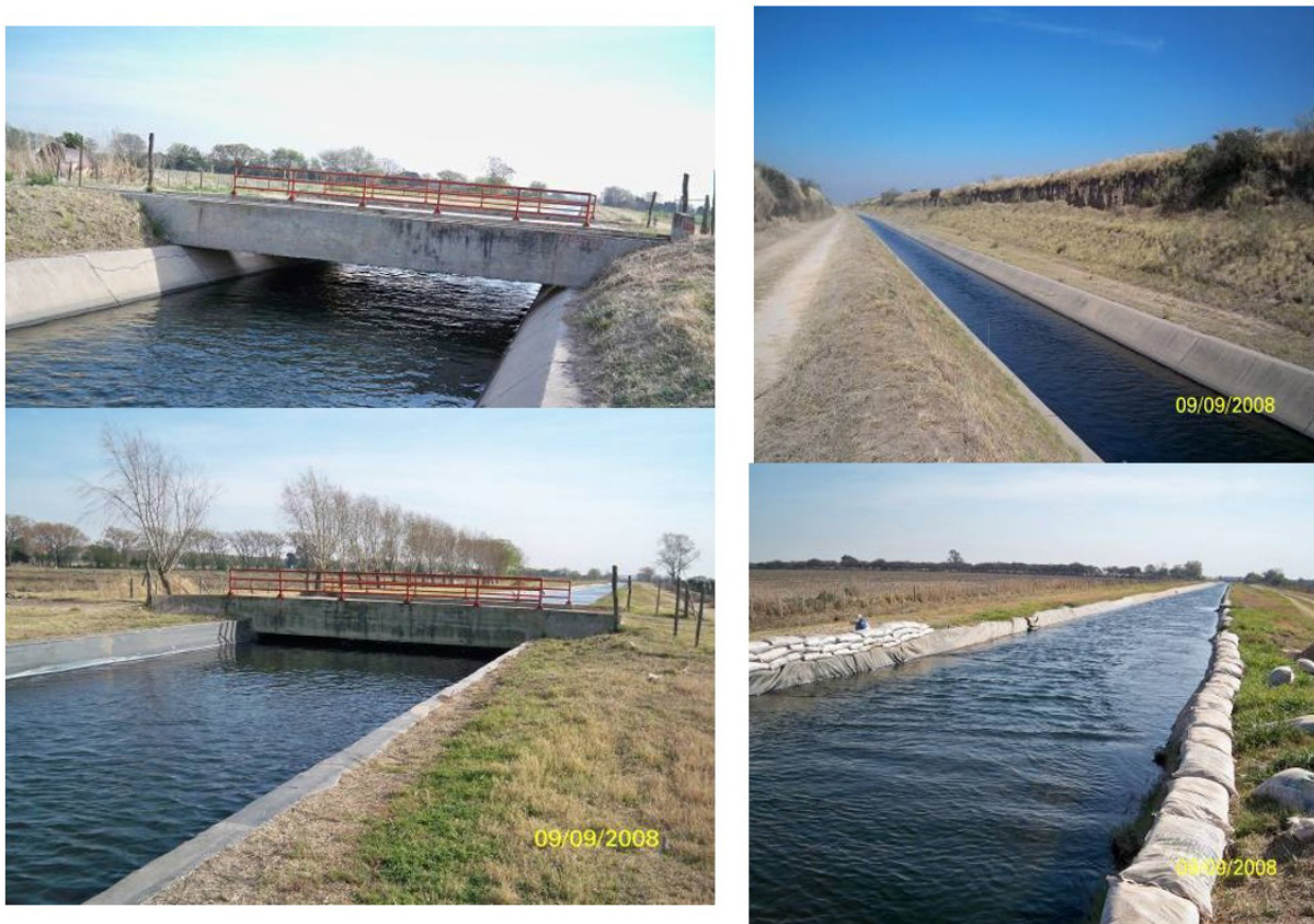
Figure 20. Bridge and Canal views before and after settlements (Terzariol, 2012).
