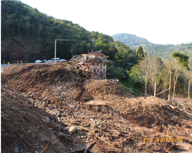
Figure 44. Landslide on slopes of Rio das Antas, near the BR470 bridge (Cleber Floriano).
