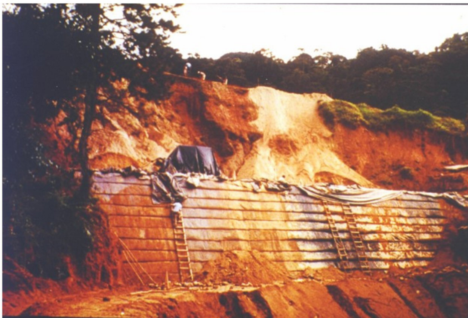
Figure 3. Geotextile reinforced slope in highway SP123 (Carvalho et al. 1986).
