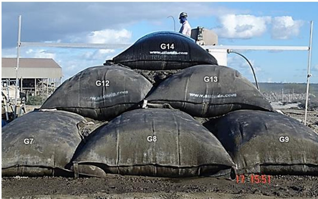
Figure 25. Stacking of geotextile tubes in the research area (Silva, 2017).
