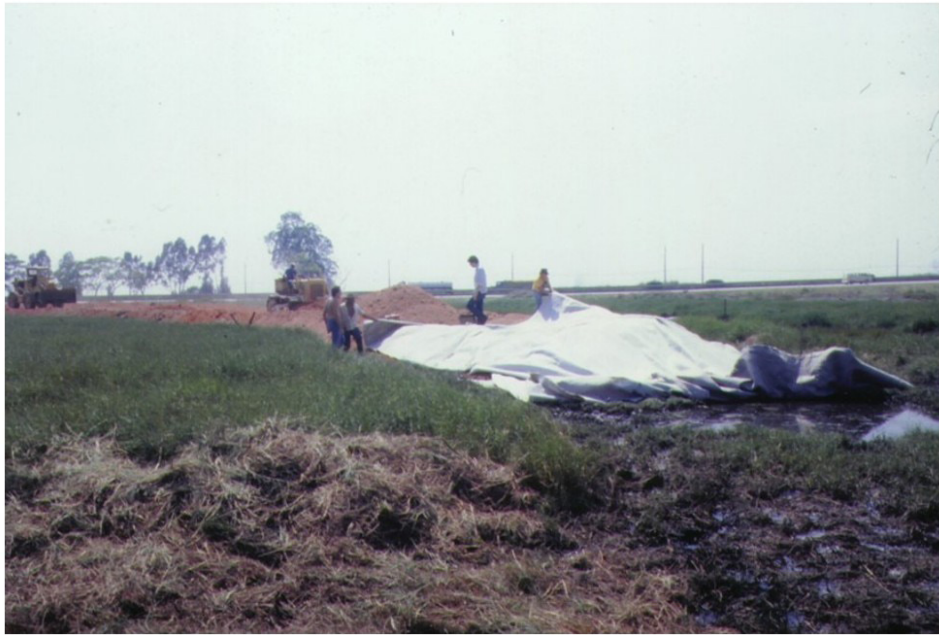
Figure 2. Pioneer research on geosynthetic reinforcement of an unpaved road on soft soil (Palmeira 1981, Ramalho-Ortigão & Palmeira 1982).
