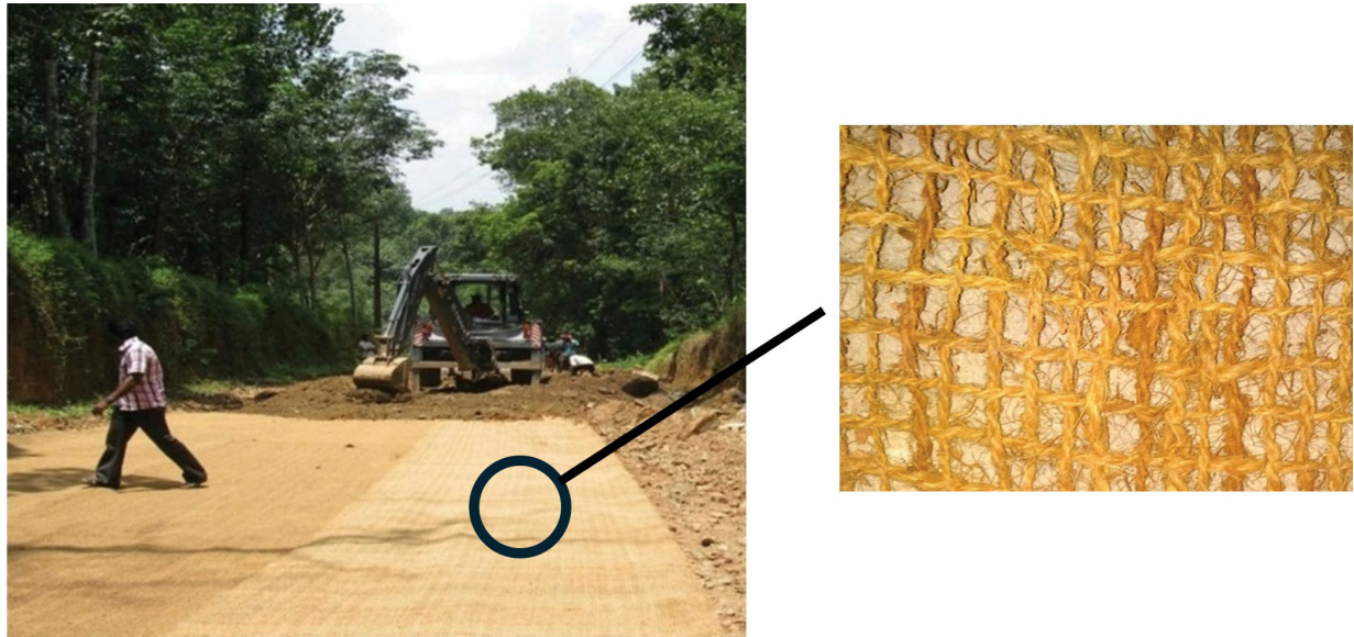
Figure 25. Coir-geotextile reinforced road during construction (Evangeline et al., 2021).
