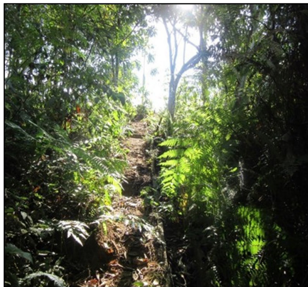
Figure 3. Dam X's downstream slope covered by vegetation, in 2015.
