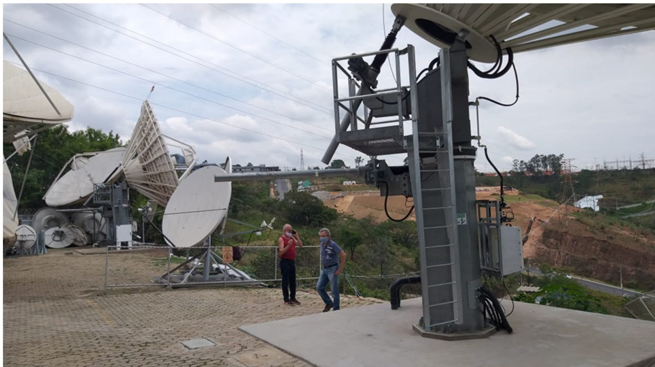
Figure 5. Overview of the antennas situated at the top of the failed slope.
