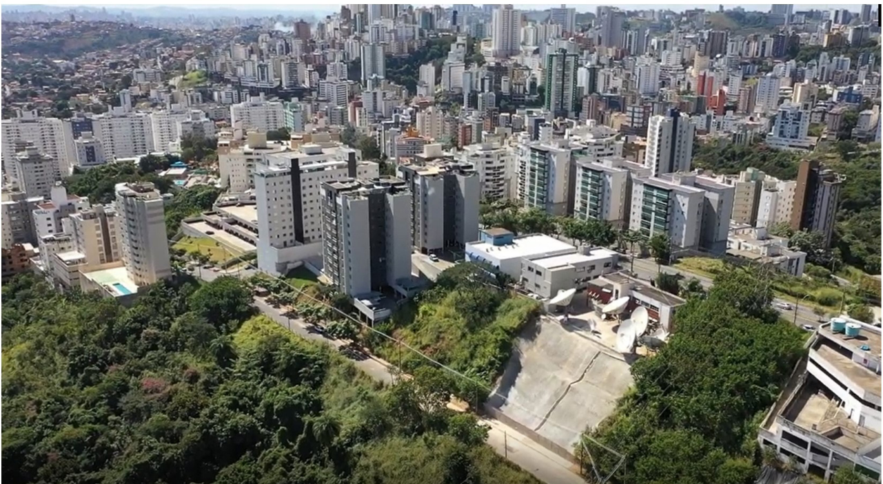
Figure 18. General view of soil nail technique and 'Buritis' neighborhood.
