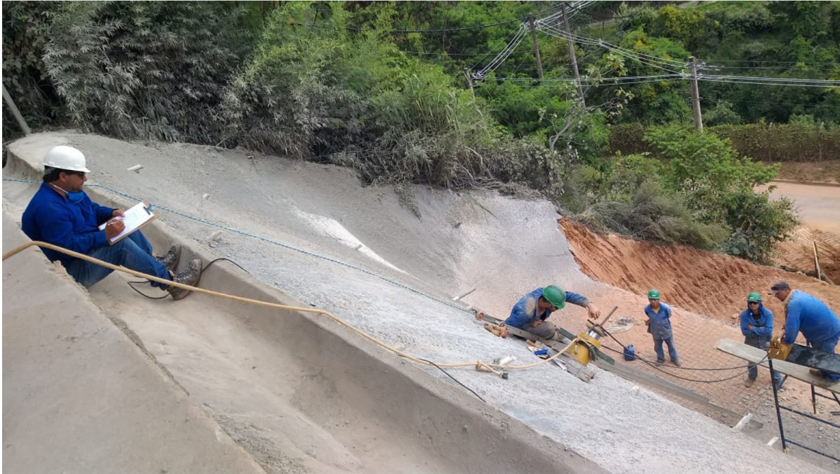
Figure 15. Performance of nailing's tensile test.
