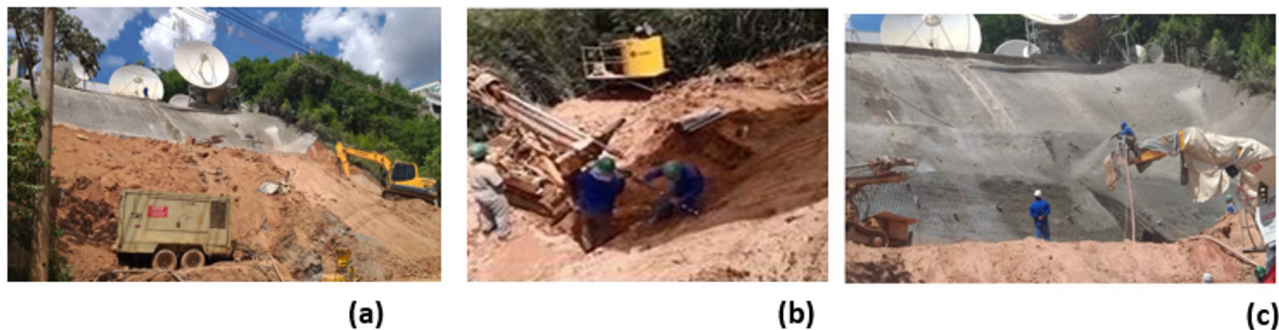
Figure 14. Phases of soil nailing execution: (a) partial Excavation; (b) Drill nail hole; (c) execution of permanent cover (including shotcrete, bearing plate and washer).
