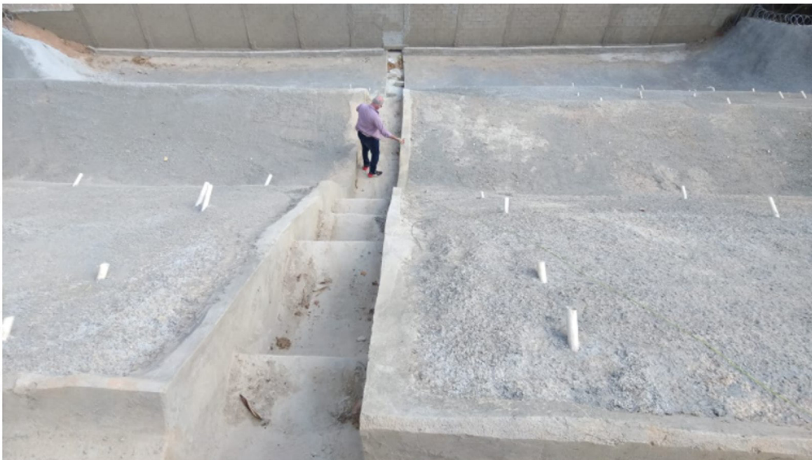
Figure 16. Completion of drain system.
