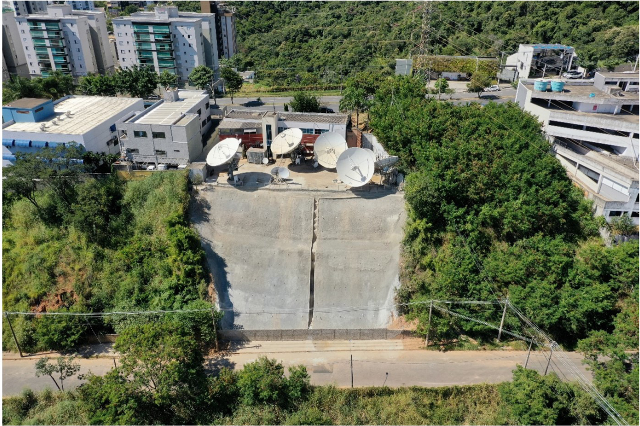
Figure 17. Front view of Soil nail technique.
