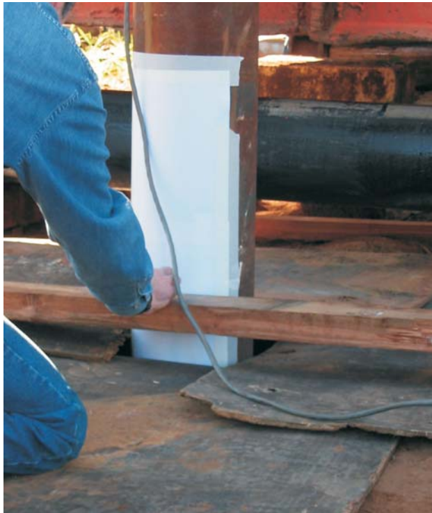
Figure 7 - Settlement measurements using paper sheet and pencil.
