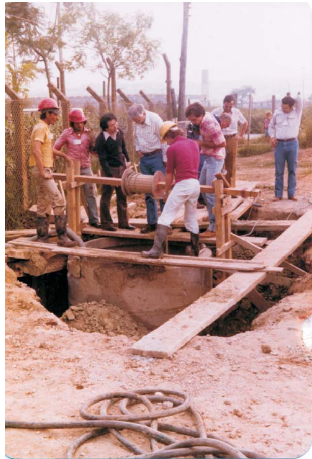
Figure 11 - Trial shaft for the River Tietê tunnel.
