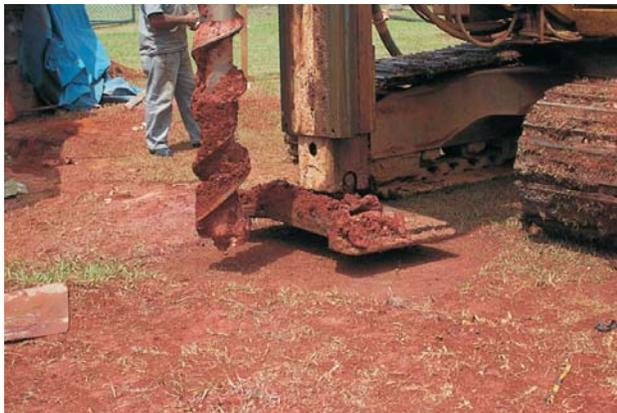
Figure 3 - CFA drilling machine.
