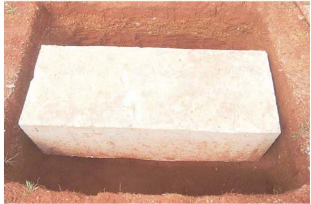
**Figure 5** - Top blocks of EHC2 and EHC3 foundations.
