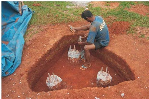
**Figure 4** - Piles of EHC1, EHC2 and EHC3 foundations before construction of the top block.
