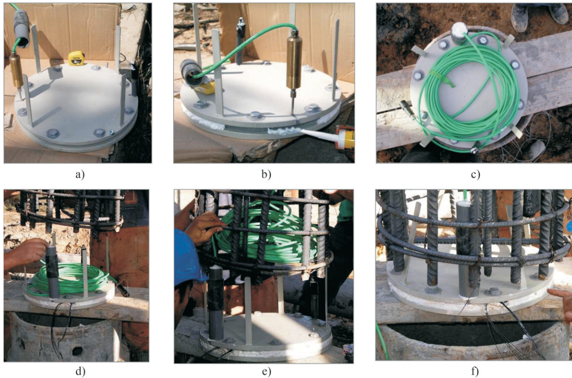
Figure 14 - Load cell installation (Costa Esteves, 2005).
