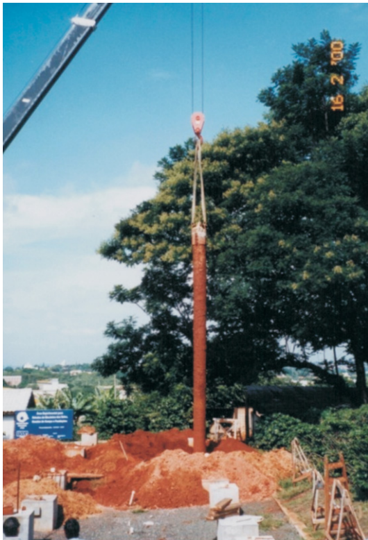
Figure 23 - Pile extraction.
