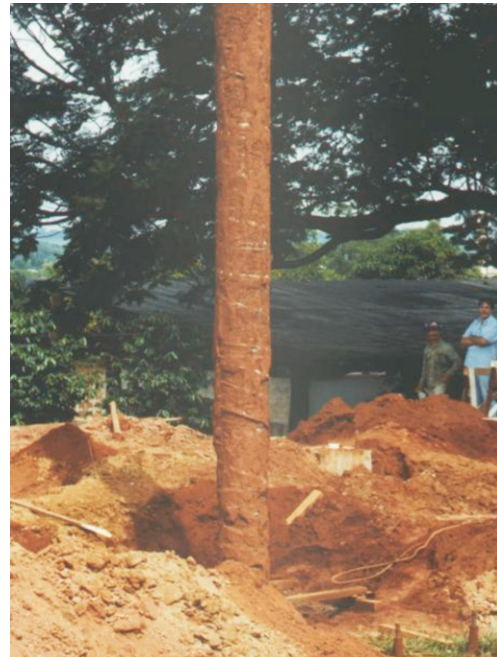
Figure 30 - Soil adherence in shaft of Omega 2 pile.
