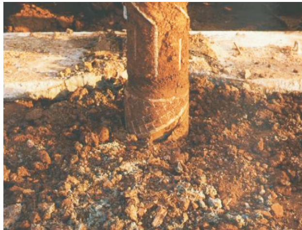
Figure 15 - Omega pile drilling.
