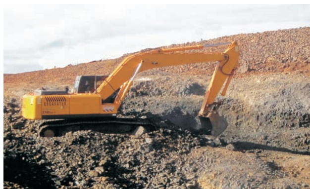
Figure 9 - Machine excavation of blocky, partially weathered entablature. São Paulo State.
