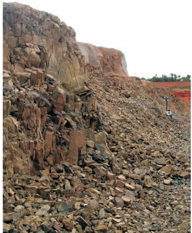
Figure 4 - Slope cut raveling in loosened entablature basalt.
