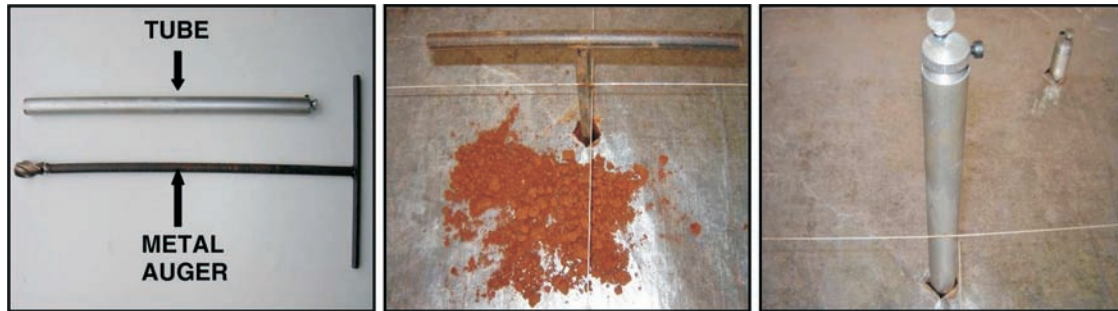
Figure 11 - Installation of monitoring tubes.
