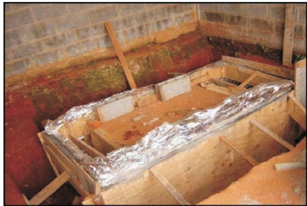
Figure 7 - Side cement walls.
