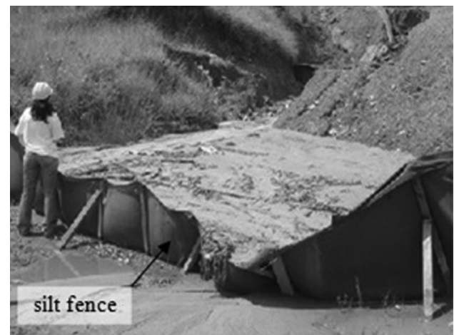
Figure 7 - Silt fence damaged due to the excess of sediment and the unsatisfactory maintenance (2 nd BMP at drainage exit # 5).
