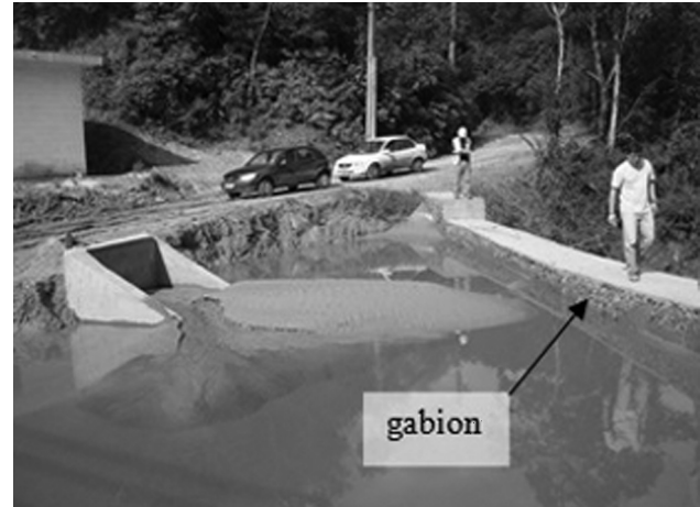
Figure 6 - Material accumulated behind the gabion (1 st BMP) at drainage exit # 4, almost overtopping it.
