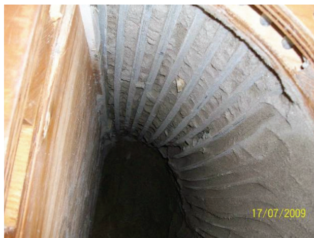
Figure 6 - Photograph of the inner part of the tunnel after excavation and application of the overload on the surface (step 5). It is possible to observe that a local arch is created between adjacent reinforcing elements, preventing material flowing.
