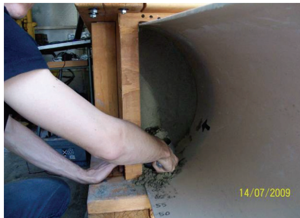
Figure 5 - Tunnel excavation by hand.
