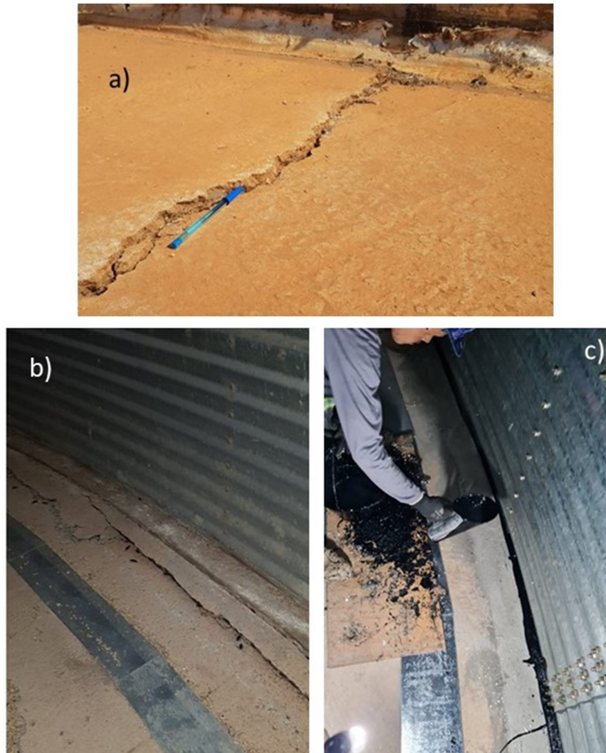
Figure 1. (a) Crack in the raft foundation; (b) structural joint opening between the raft and the beam ring; (c) sealing of the joint after opening.
