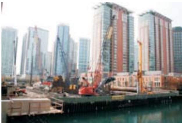
Figure 20 - Beginning of excavations for the Chicago Spire foundation.
