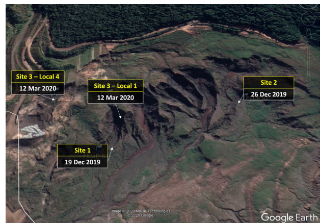
Figure 3. Location of the three sampling sites on B1 dam, after failure.
