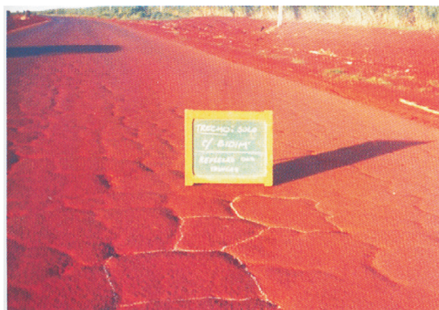
Figure 3 - Cracking on pavement made of fine and coarse lateritic soils (Villibor, 2009).
