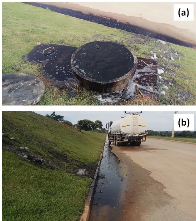
Figure 4. Leachate leaks: (a) gas drainage with leachate; (b) flow of leachate along the road.
