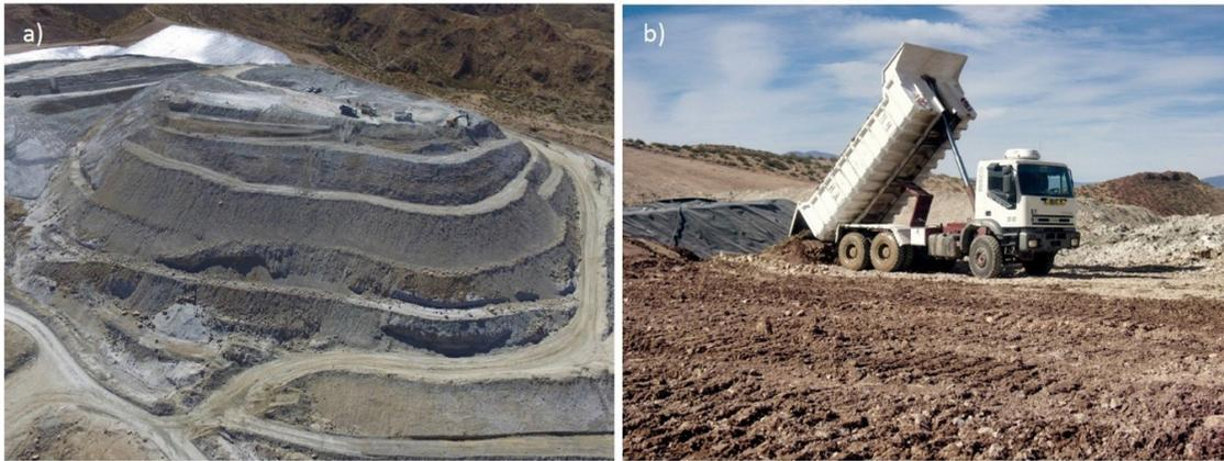
**Figure 1.** (a) Stack of filtered tailings under construction. Casposo Mine, San Juan, Argentina (Photo: courtesy of Casposo Argentina, published with permission); (b) Tailings transport and distribution with conventional earthmoving equipment requires achieving trafficability.
